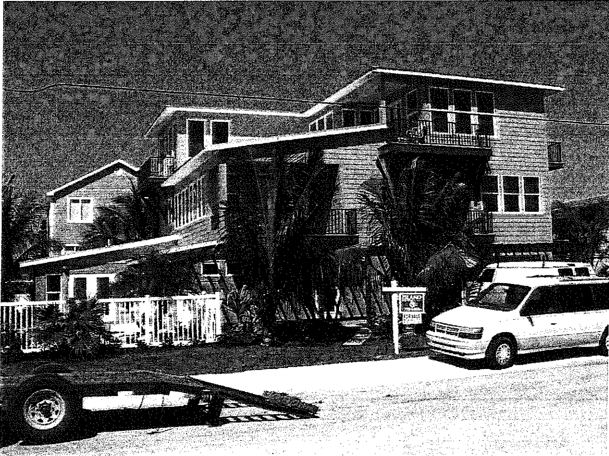
VIEW FROM SOUTHWEST - UNIT 'A' NEAREST 100 52nd STREET HOLMES BEACH, FL
